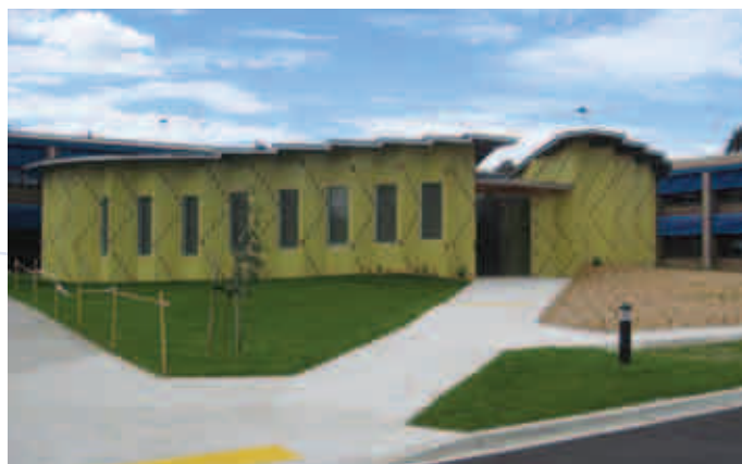
New Administration Building
